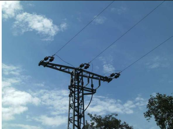
*Fig. 1.2-2: Steel grid pylons with double (redundant) strain-type (horizontal) insulators, in Germany commonly in use. They are grossly underestimated “killer poles”. (photo: Haeusler)*
