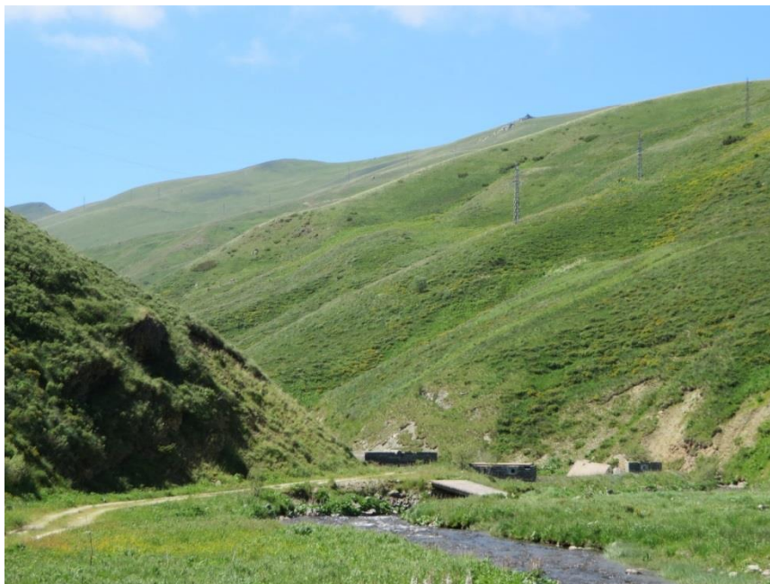
Figure 1: The crown of the dam would be located between the lower and the second pole (⇔) of the electric line on the right-hand slope, with the crown stretching across a length of 335 m. © R. Brunner
