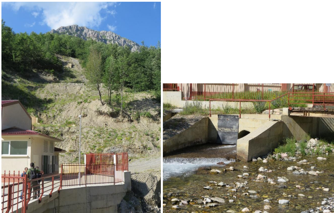
Figure 6: Left: Small HPP near Tresonce. The pressure pipe runs under the sandy slope. Right: The outlet of the small HPP (left) and the river with a reduced discharge (right). This HPP is located inside the National Park Mavrovo. © R. Brunner
