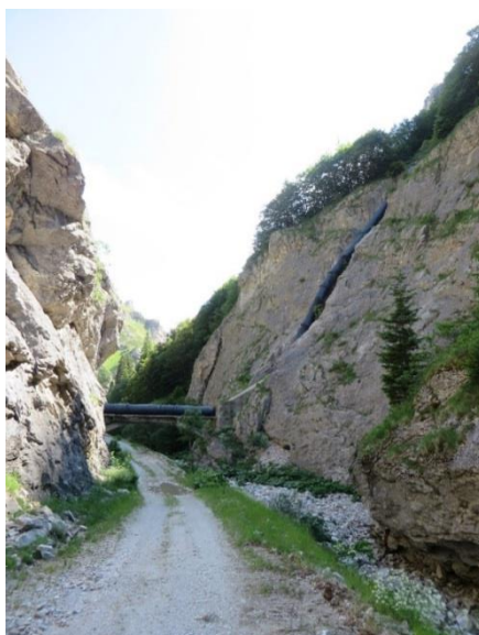
Figure 3: An existing steel siphon would be integrated into the HPP system. The picture also shows the present state of the access road to the Lukovo Pole site. The Radika riverbed on the right is dry. © R. Brunner
