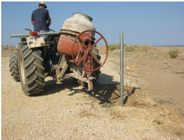
Photo 15: Pouring concrete in the sand dune zone for the installation of the traffic bars (proved unsuccessful).
