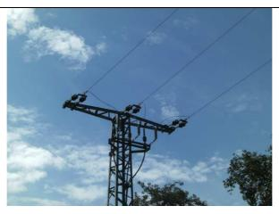
Fig. 1.2-2: Steel grid pylons with double (redundant) strain-type (horizontal) insulators, in Germany commonly in use. They are grossly underestimated "killer poles". (photo: Haeusler)
