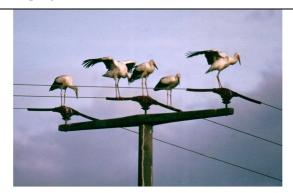
Fig. 1.2-1: Insulating hoods for upright (pin-type) insulators - a success story in Germany (photo: Walter Feld)
